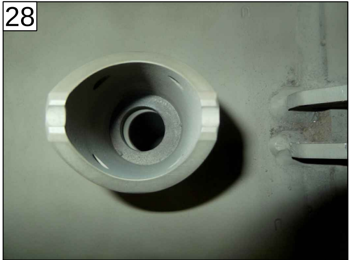
LINE UP LOCK-PIN HOLES FOR PULLOUT & CROSSTUBE
