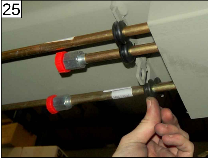
PUSH GROMMETS AROUND TUBES PAGE 21 - ITEM 24
