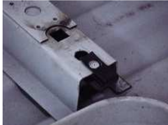
Fig 2 - U-nut Installation
